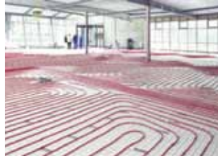
Radiant Heating and Cooling
